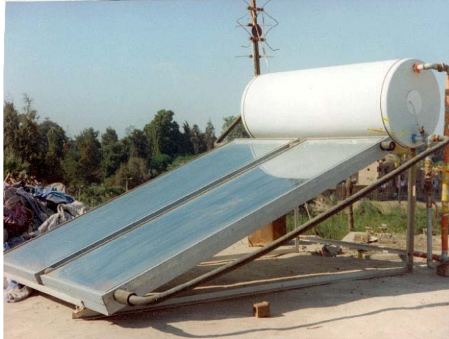
Image W-i 13: Solar thermal water heating system.
